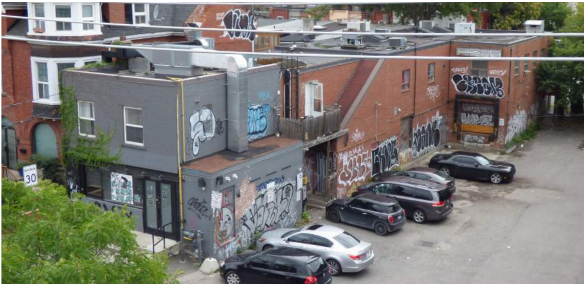
8. View of the north (principal) and west elevations of 17 St. Andrew Street, looking southeast from the above-grade parking structure on the north side of St. Andrew Street.
