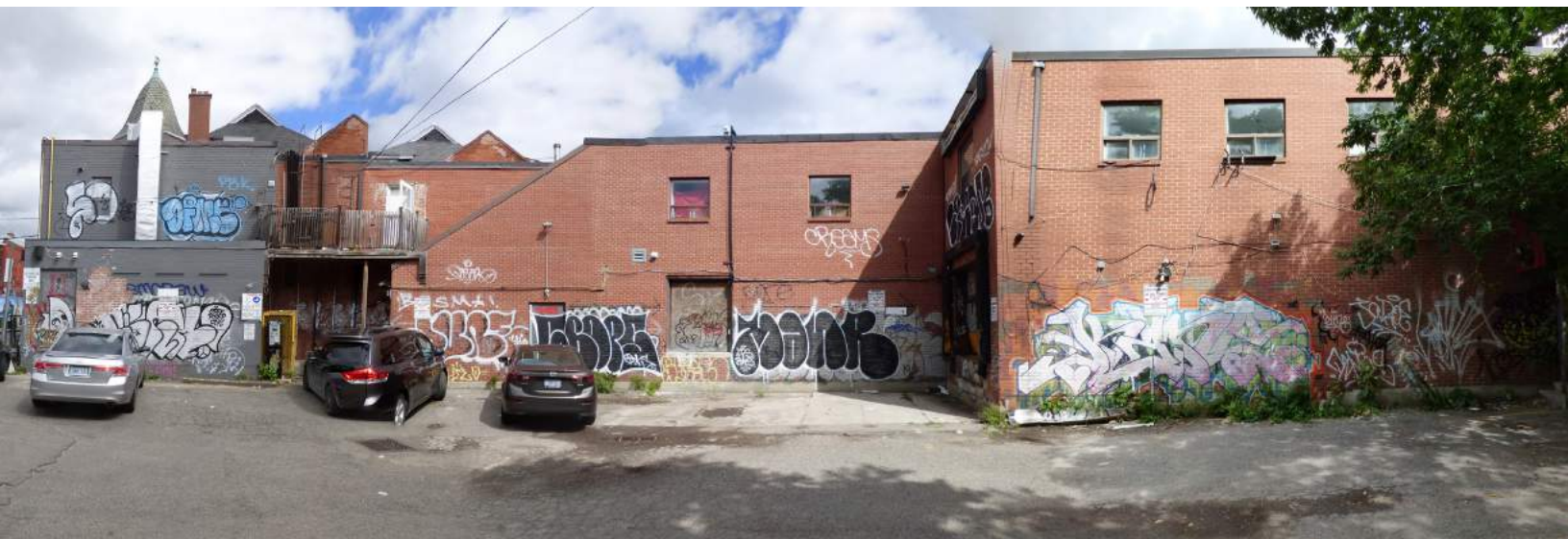
3. West elevation of 17 St. Andrew Street.
