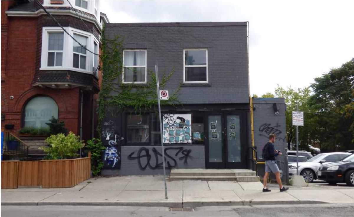
2. North elevation of 17 St. Andrew Street.
