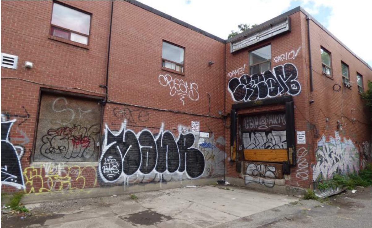
4. North return wall at the west elevation of 17 St. Andrew Street.
